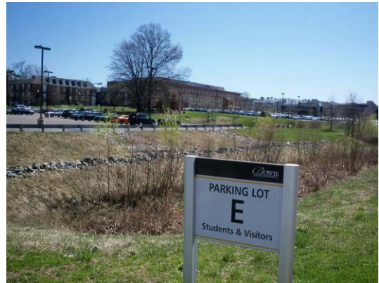
Typical storm water mgt near west parking lots
