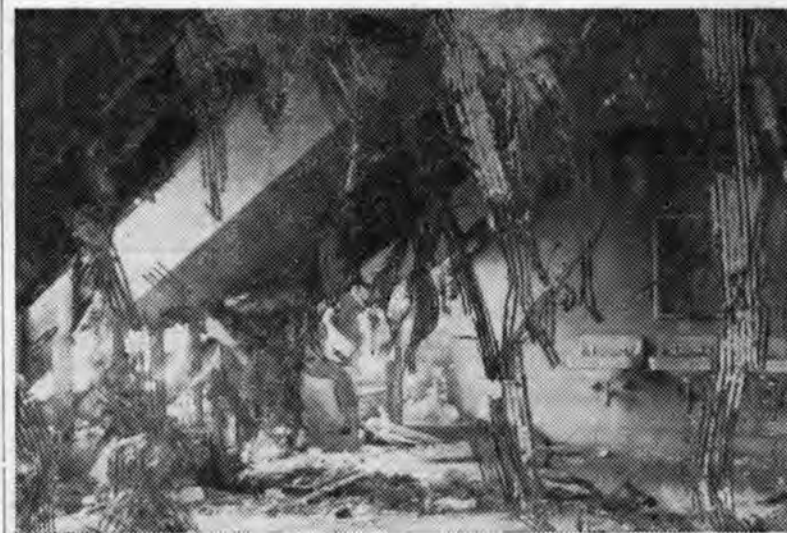
Mr. Stanford, campus photographer, took this picture of a section of the third floor of Tubman Hall, depicting the extent of the damage wrought by the fire.
